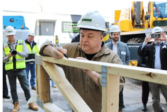
Cambridge Vice Mayor Marc McGovern signs beam
