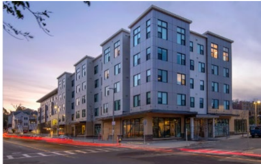
BARTLETT STATION, BUILDING B
