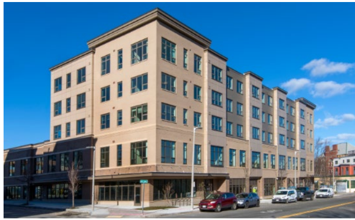
BARTLETT STATION, BUILDING A
